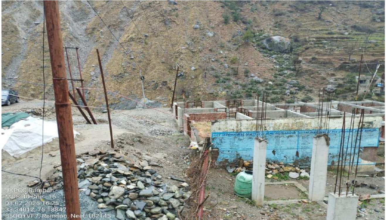
The site stabilized and closed.
