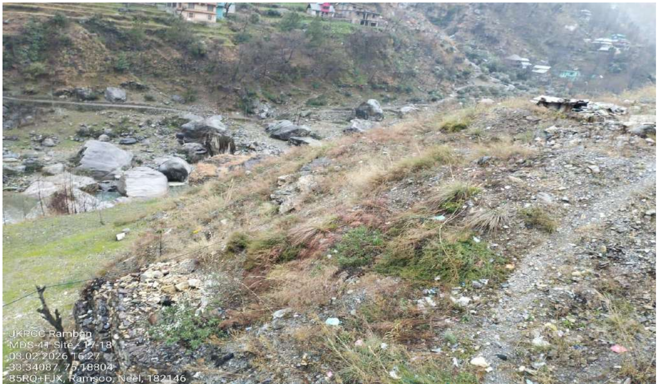
The site stabilized and closed.
