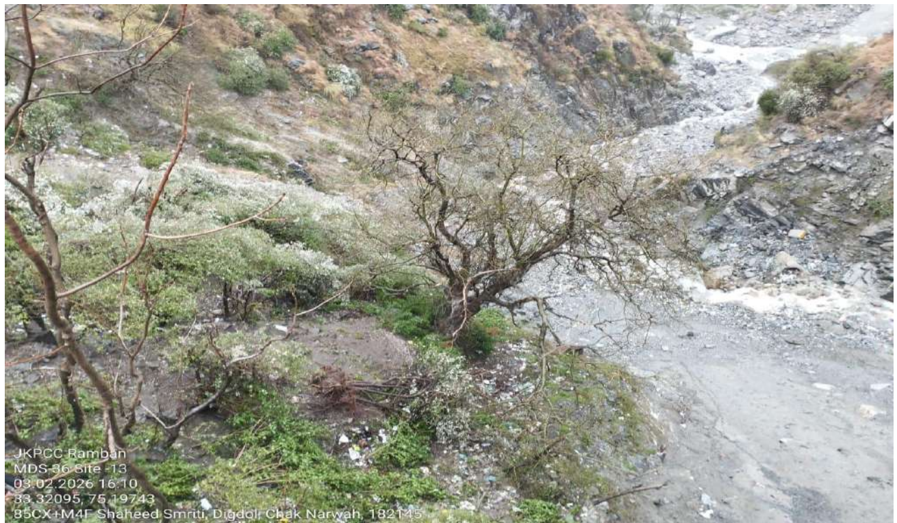
The site stabilized and closed.
