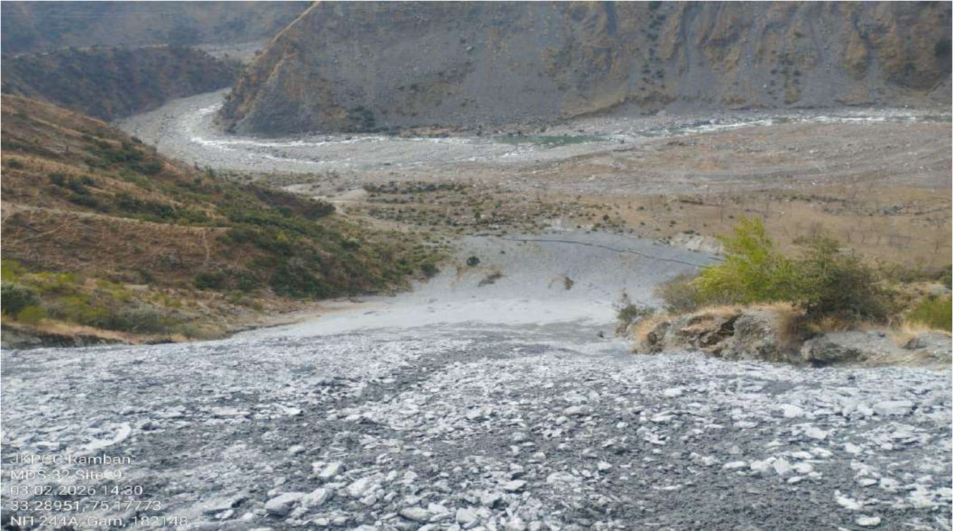
Site is operational needs to provide protection as dumping progresses.
