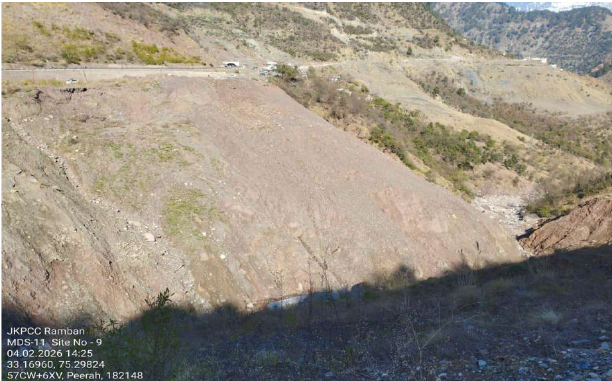
Needs to provide gabions / protection along nallah in washed away stretch.
