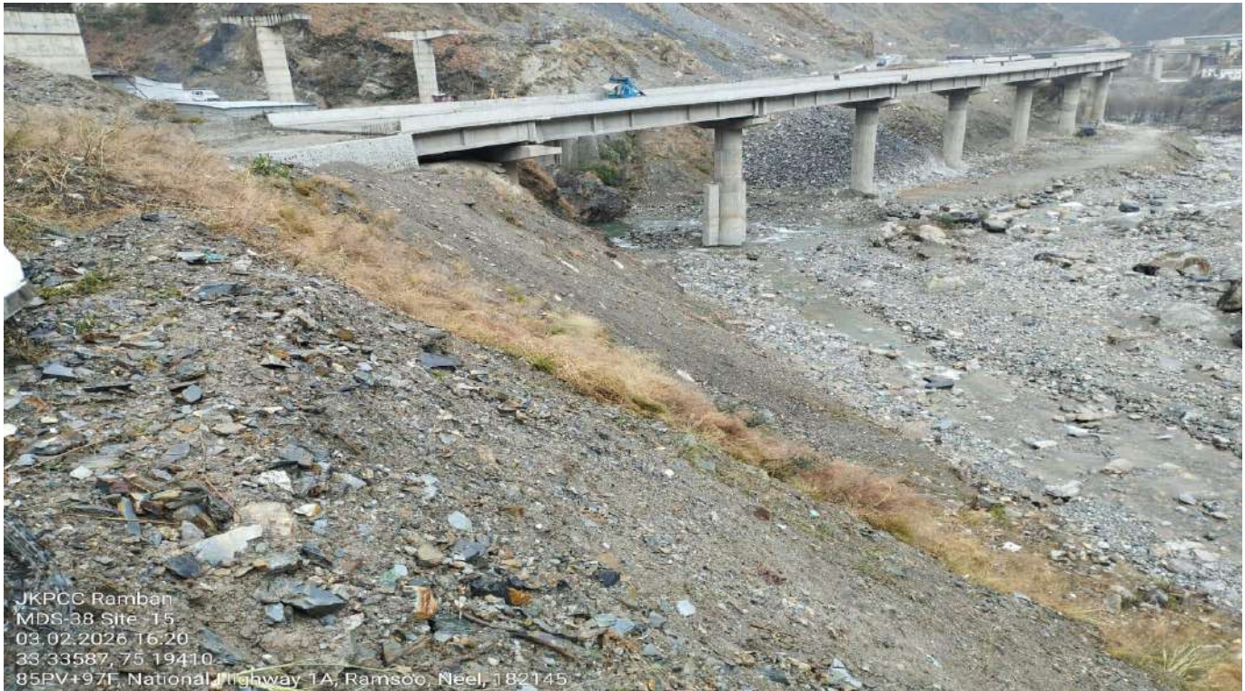
The site stabilized and closed.
