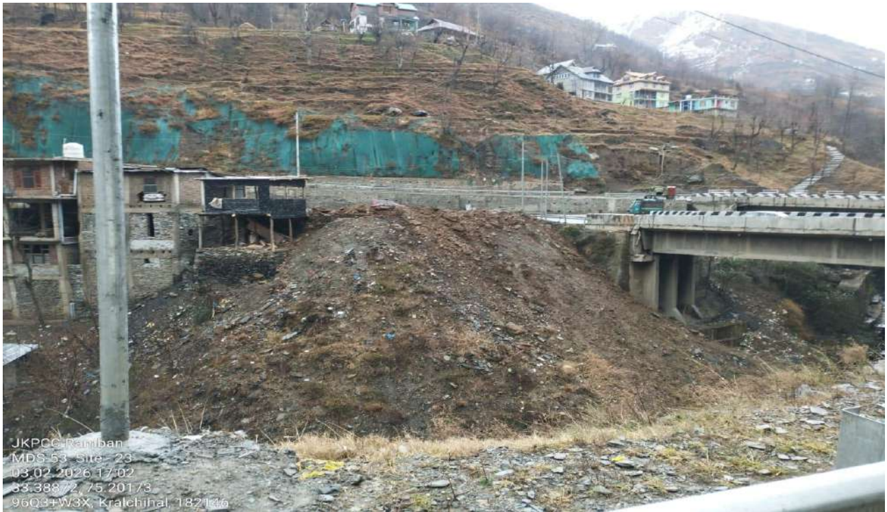
The site stabilized and closed.
